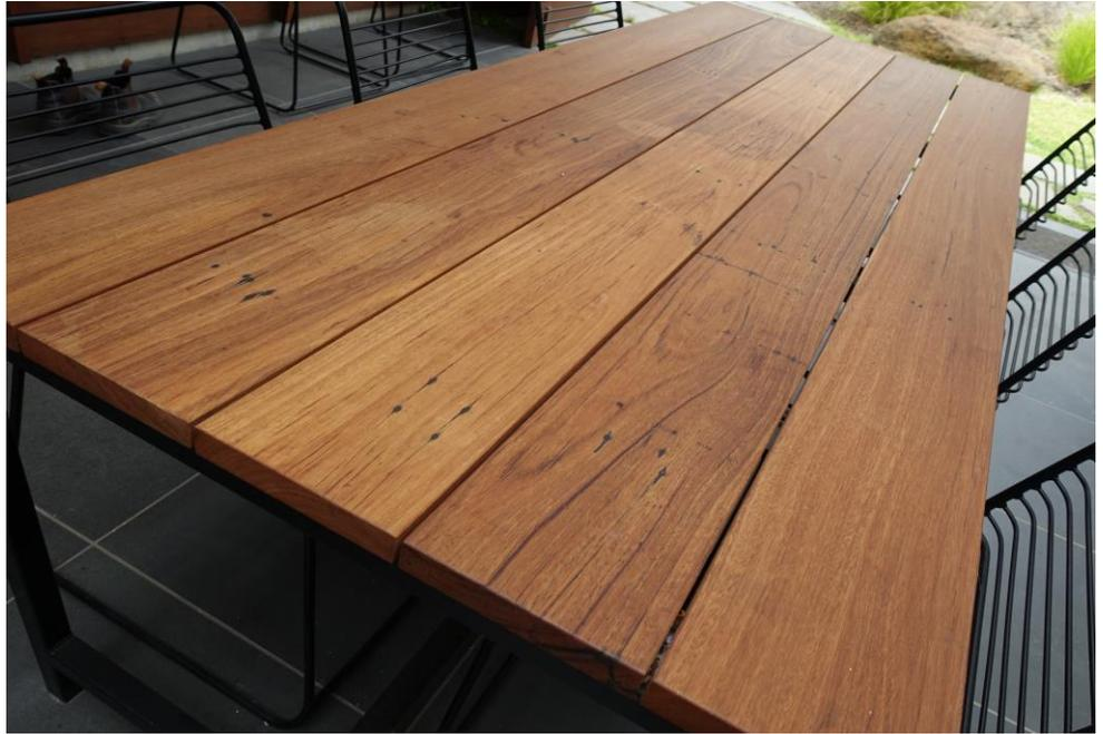
Arissed edged Recycled Messmate boards with 3mm gap on covered courtyard table
